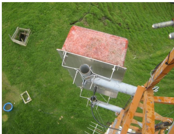
Panel UHF Vértice 3 a 27m
