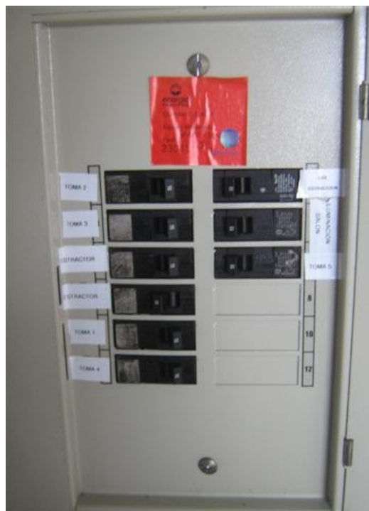
d tablero general de breakers
