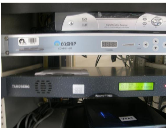
Receptor satelital de radio
