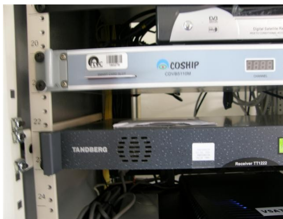
Receptor satelital de radio
