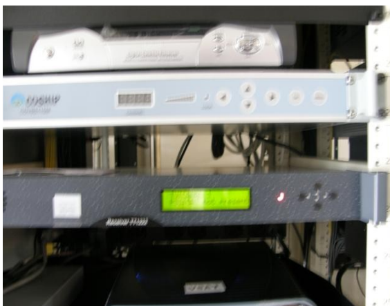
Receptor satelital de radio
