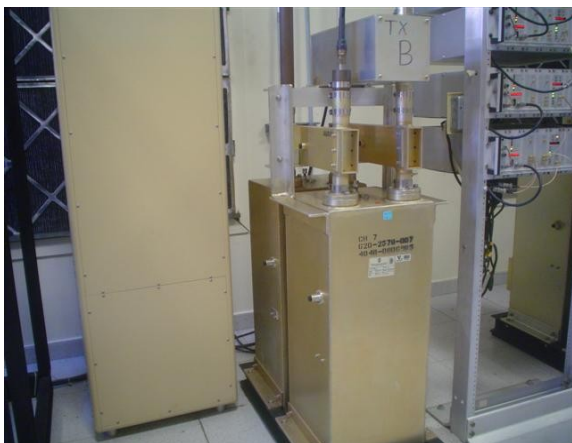
Diplexor B Transmisor Principal Canal Uno
