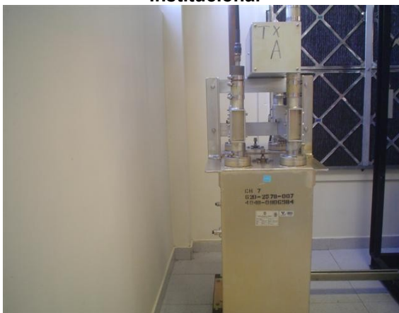
Diplexor A Transmisor Principal Canal Uno
