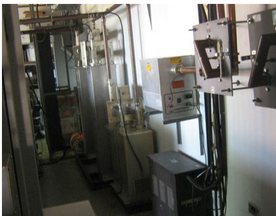
transferencia red- carga fantasma TX Harris Radionica
