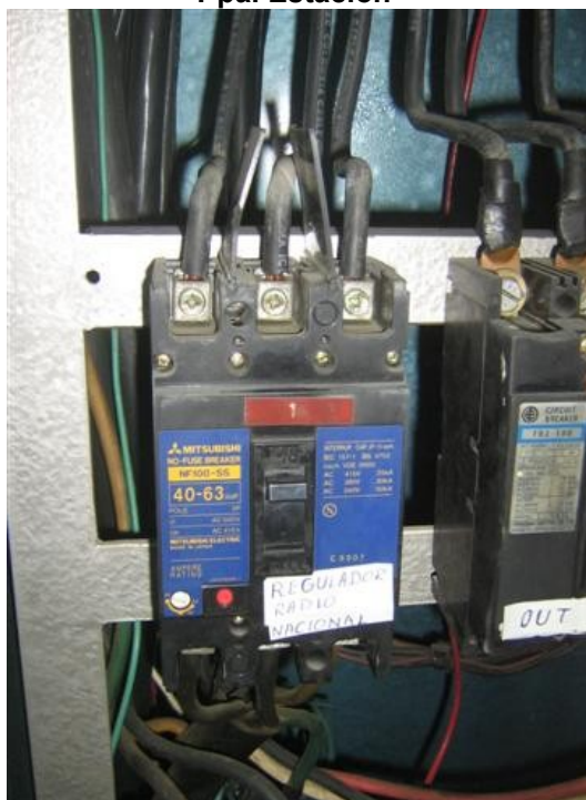
Breaker Ppal TX Radionica
