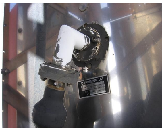
Conector antena
