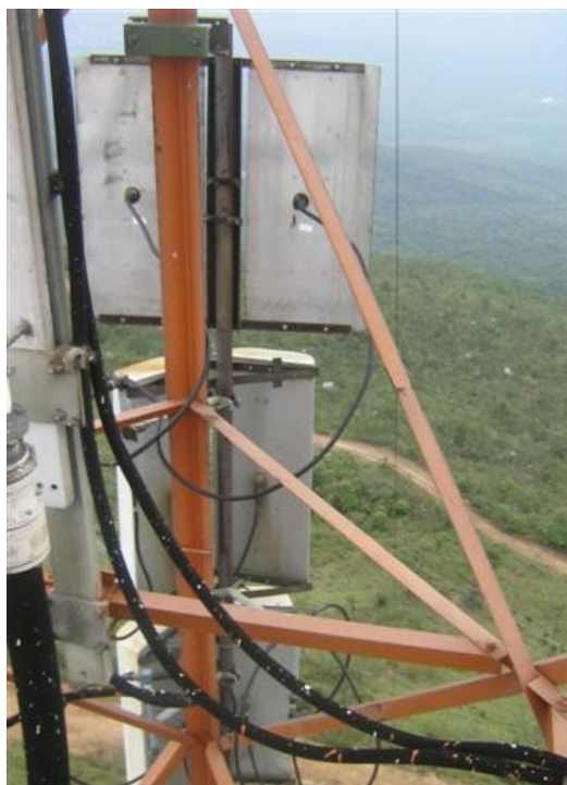
Antena panel UHF torre 1
